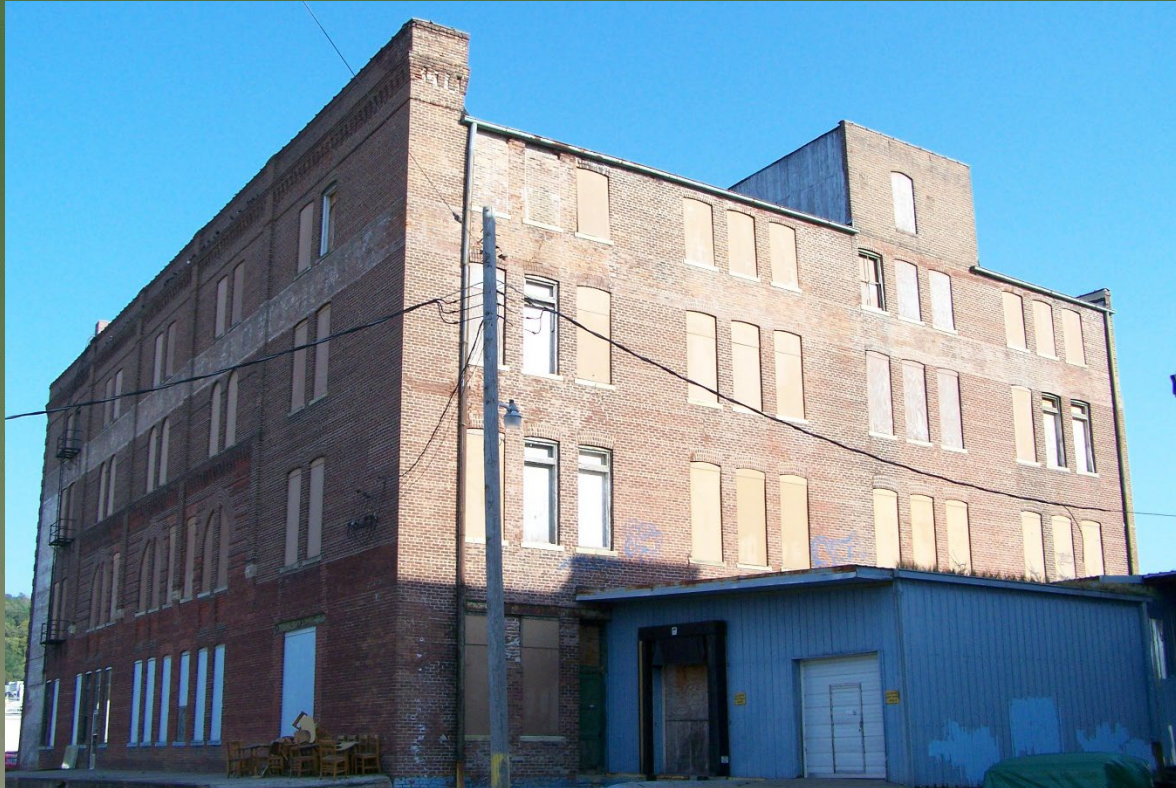
1888 Construction – Next to Railyard
