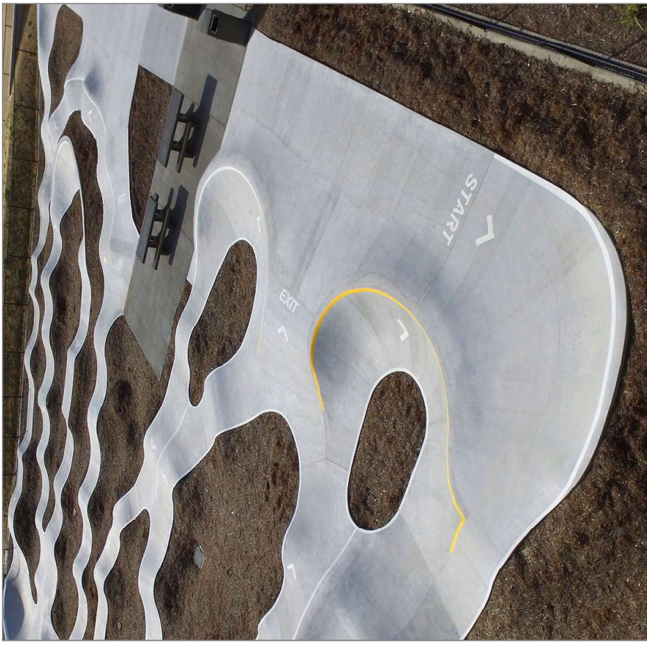
Pump Tracks ( https://www.spohnranch.com/portfolio/pacific-highlands-ranch-pump-track )
