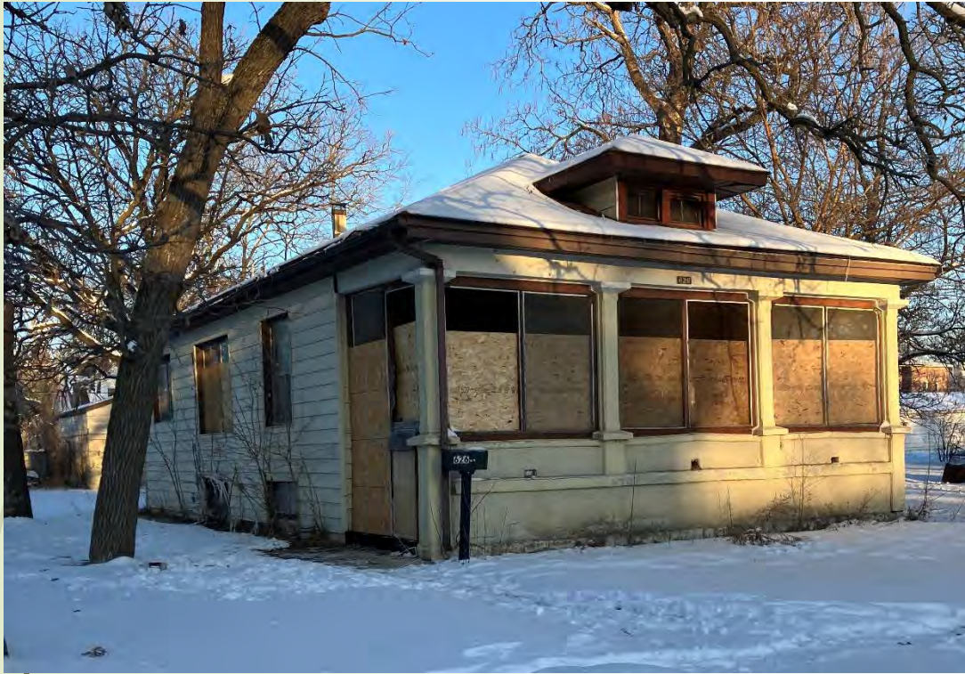
626 North Delaware Avenue
